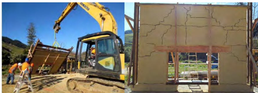
Figure 2: Adobe veneer wall panel 4m x 3m with lintel, a) tilt test at about 45 degrees, b) highlighted crack pattern following all tests. Photos: Hugh Morris
