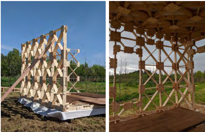
Figure 2. Wall Frame and Sub-Floor during Assembly
