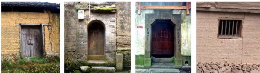
Figure 10: Door and Window Openings on Rammed Earth Wall
