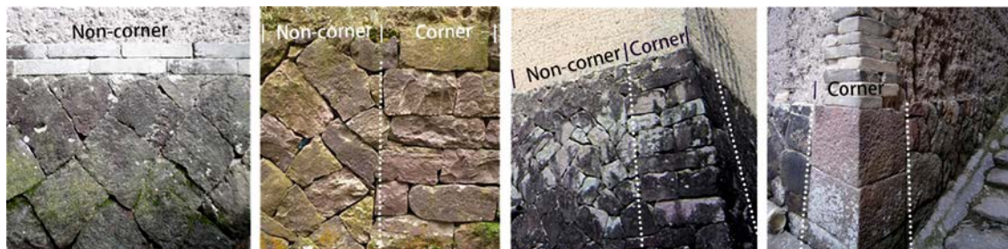
Figure 2: Stone foundation types
