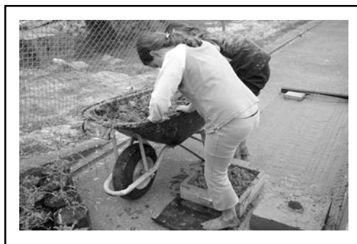
Fig 3: Students making clay bricks for one wall.
