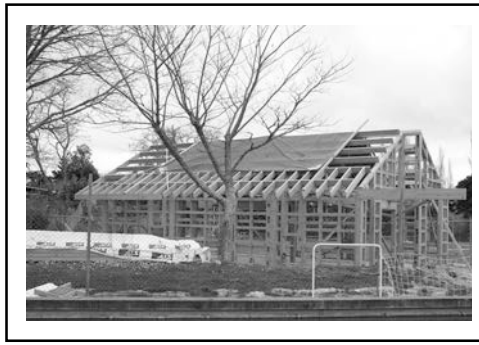
Fig 1: Eco-classroom under construction. Sept 2009
