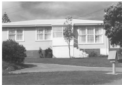
Figure 2: Austrian Prefabricated House Titahi Bay, Wellington NZ. Contractor: Thermo Insulated Units Ltd.
