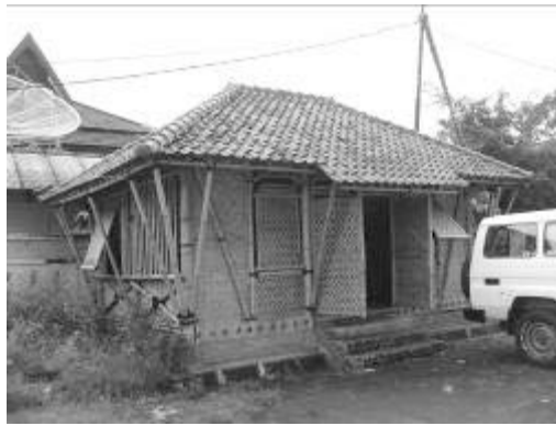
Figure 1: Bamboo transitional shelter in Yogyakarta
