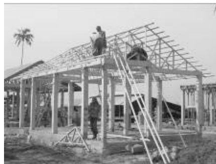
Figure 3: Caritas reconstruction house under construction (source: Ingvar Ando)
