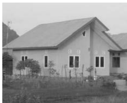
Figure 4: Reconstruction house built by Habitat (source: Wing Roharjo)
