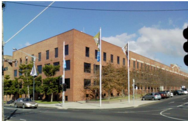
Figure 2: Deakin University's Waterfront Campus Building.
